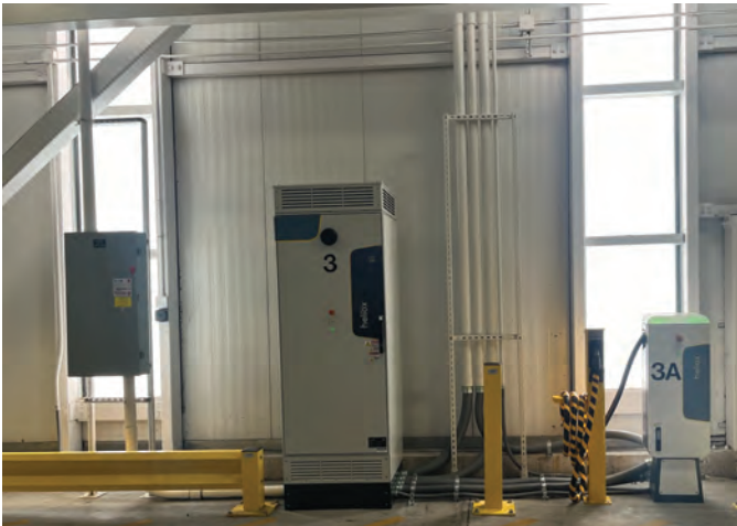
Phase 1 New Charging Station Installation at Cottage Street, Springfield
